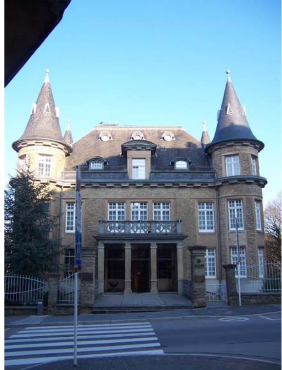
Ministry of the Interior
