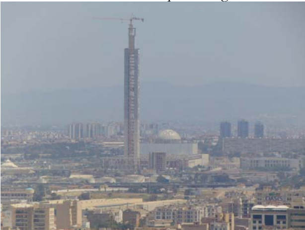
The New Mosque in Algiers (under construction)
